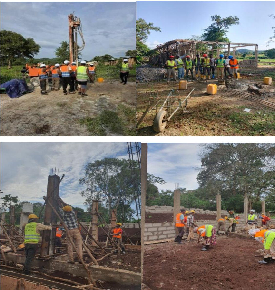
Fig 11 : Buldigilu drilling of SW, construction of of schools at Bullen, Mao-komo special woredas.
