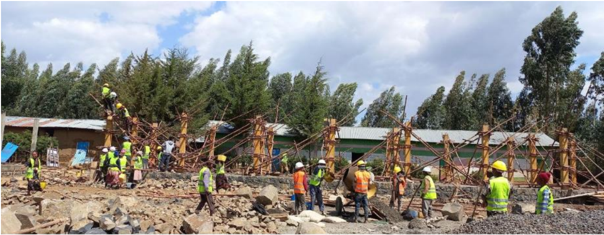
Fig 10: Construction in Meket, Amhara Region.
