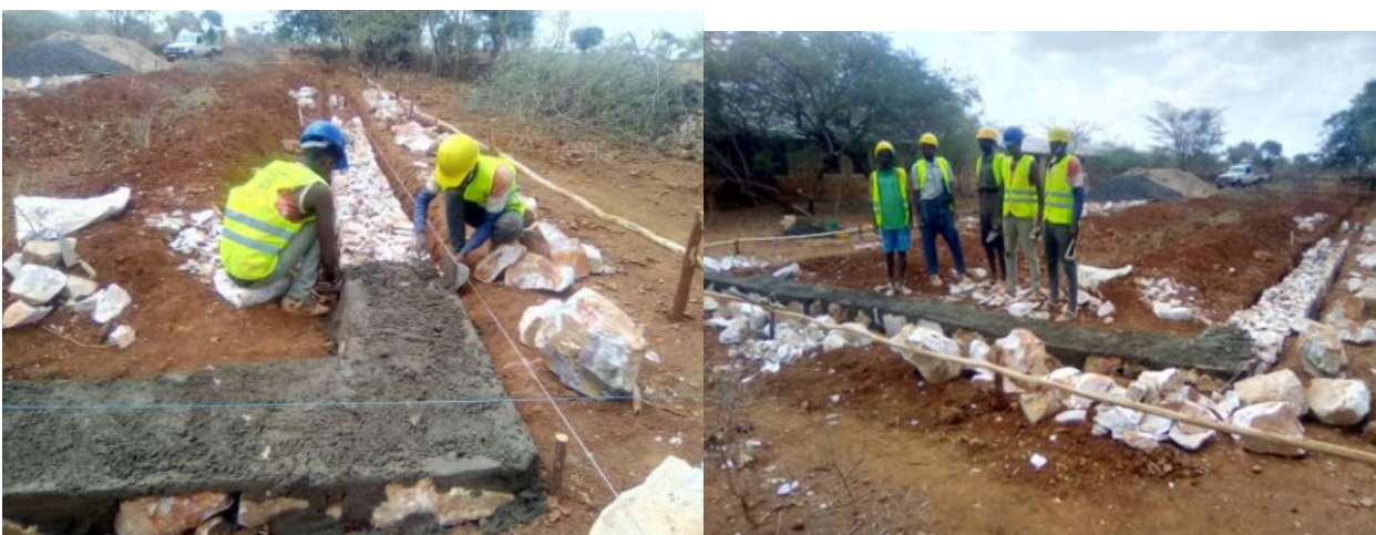
Fig9: Tigray Region, Woreda Seharti, construction site (Sample photos)
