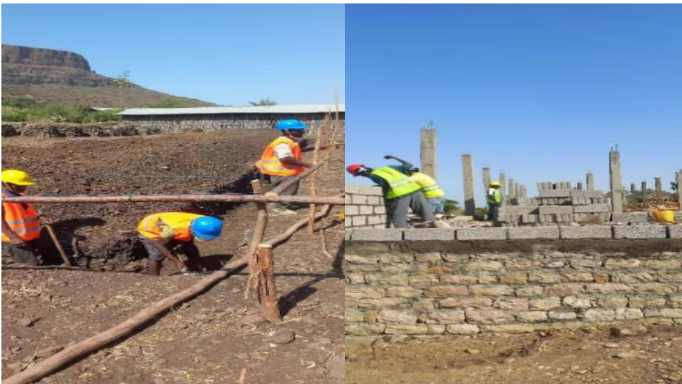
Fig8: Tigray Region Woreda, Emba Alaje construction site (Sample photos
